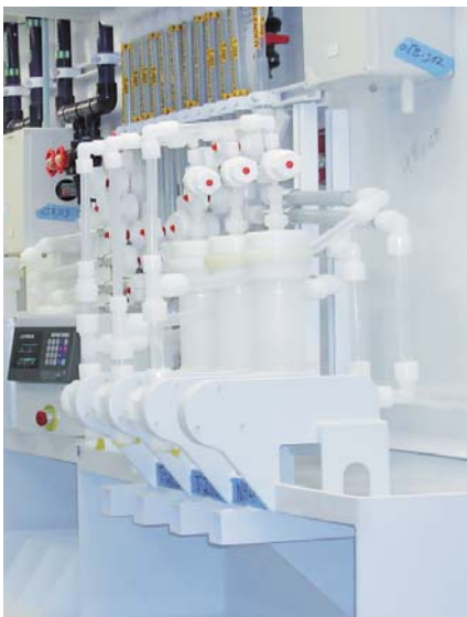
Chemical filling installation
