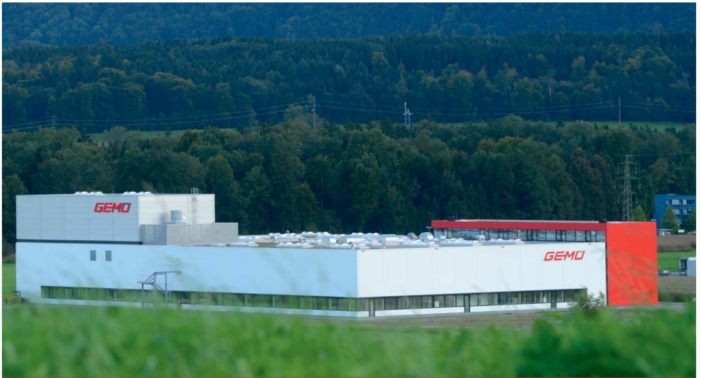
Outdoor photo of the new building in Emmen / Canton Lucerne / CH
