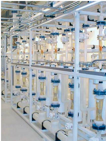
Basic supply of semiconductor factories, ultra pure water treatment
